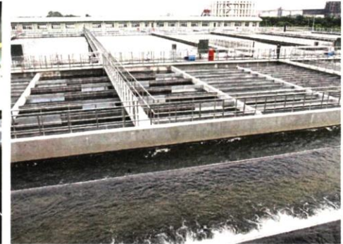
The new water treatment plant features the latest technologies used to extract, treat and distribute water.
