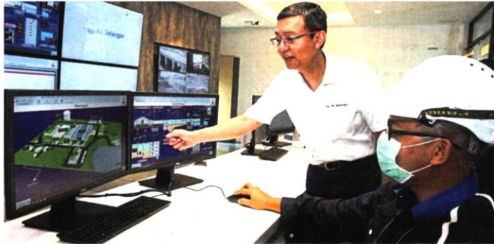
Suhaimi (left) visiting the command centre of the newly opened Labohan Dagang water treatment plant in Kuala Langat, Selangor. The plant can supply up to 200MLD of treated water to users in the region.
